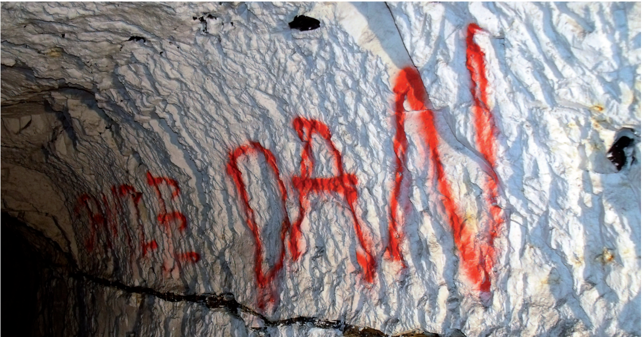
Above: Recent red paint applied on a large scale in the unlined sections of the tunnels.
