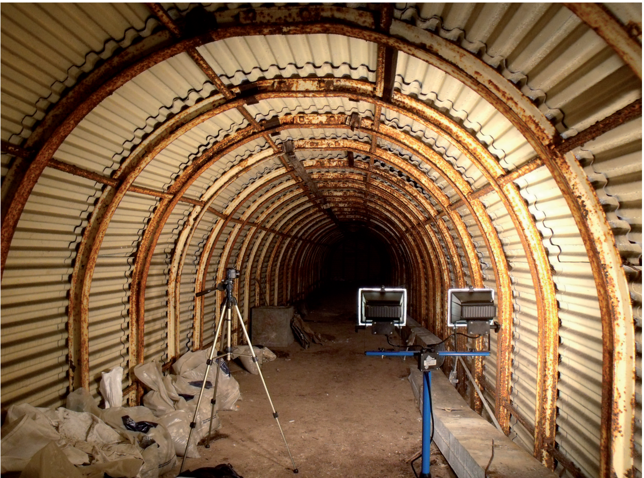
Above: Section of the northern communications tunnel, looking eastwards.
