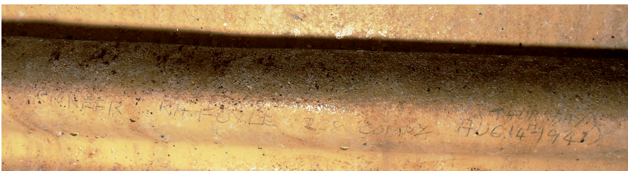
Below: Pioneer Reginald Arthur Foyle left this inscription on Thursday the 14th of August, 1941; most probably marking the completion of this section of work on the tunnels.
