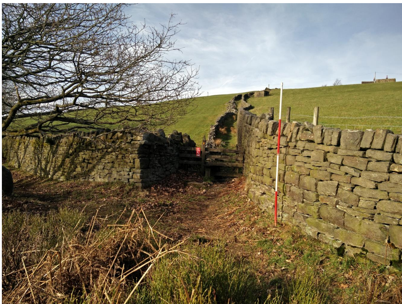
Plate 14: Gateway between Foul Scout Wood and walled lane running between fields up to Shackleton (visible in top right of photograph). The surrounding dry stone walls are post-medieval. Site FS102. Image copyright Pennine Prospects.
