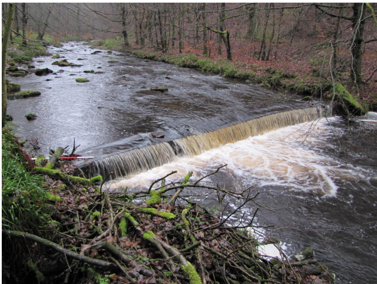
Plate 18: Weir constructed of cast iron across Hebden Water, serving a culvert taking water to one of the mill ponds above Gibson Mill (site IH04). Image copyright Pennine Prospects.
