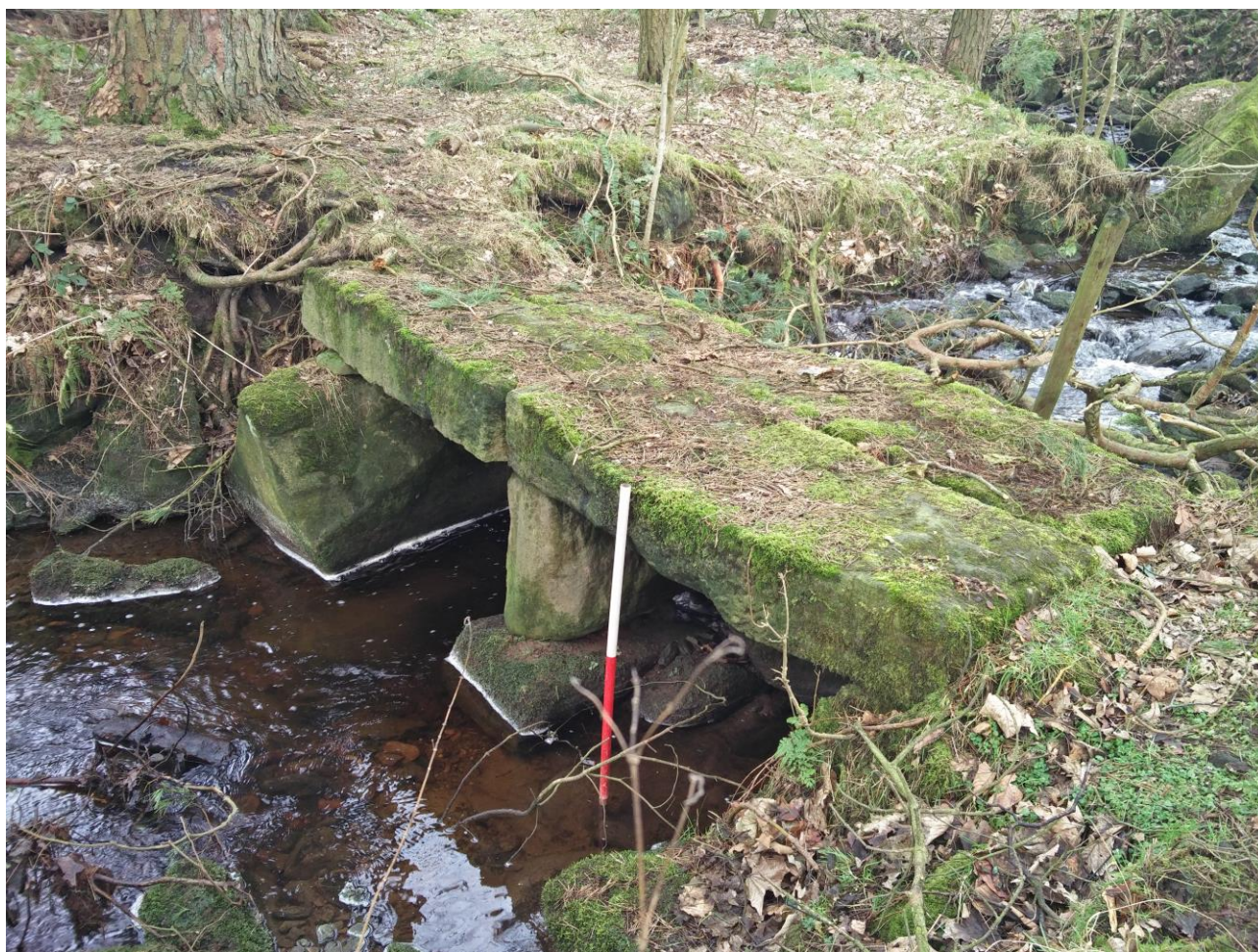
Plate 13: Stone clapper bridge at head of Rowshaw Clough, Walshaw Wood (Site FS094). Image copyright Pennine Prospects.
